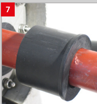
7 Insert multilayer inserts one after the other.
