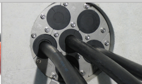
7 Insert multilayer inserts one after the other.
