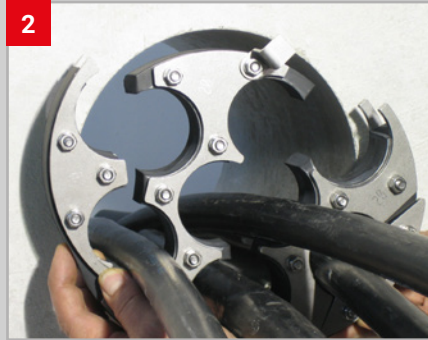
2 Remove multilayer inserts and place opened rubber press seal around the cable.
