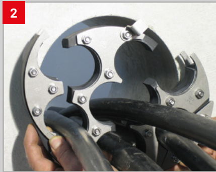
2 Remove onion ring inserts and place opened rubber press gasket around the cable.
