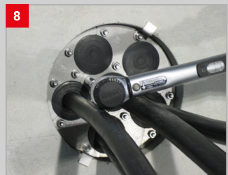
8 Tighten the nuts. Finished! Watertight up to 2.5 bar
